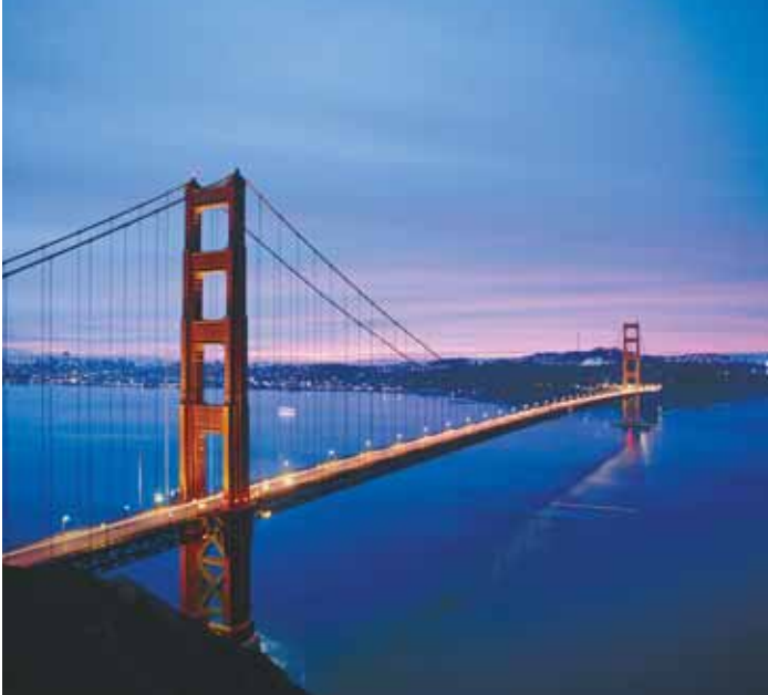
Golden Gate Bridge, San Francisco
